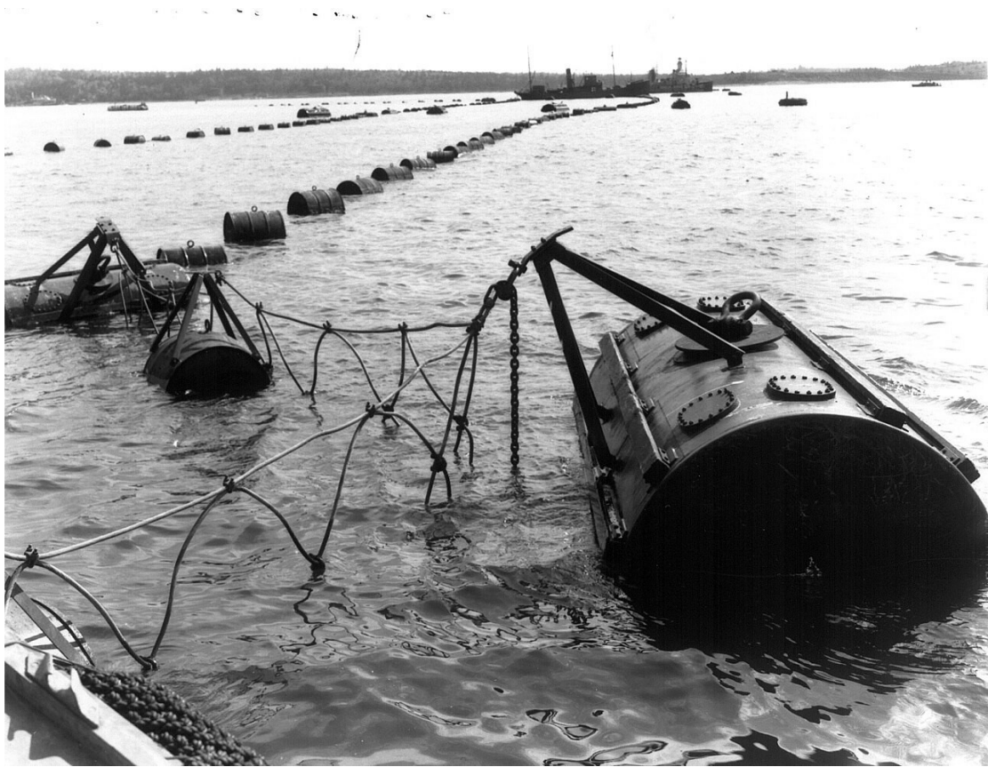
An anti-submarine net similar to what was installed in St. Lucia Source: Library and Archives Canada
